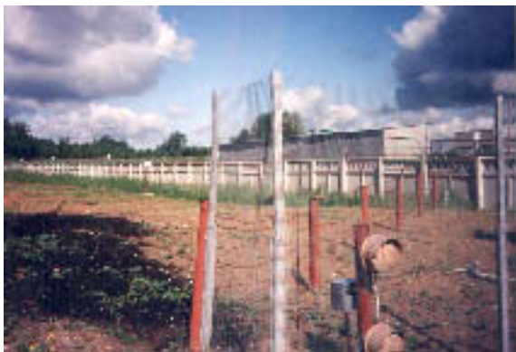
Figure 4-1: The perimeter surrounding Ignalina NPP, including some of the (later replaced) systems for physical protection (Photo: NPRA)
