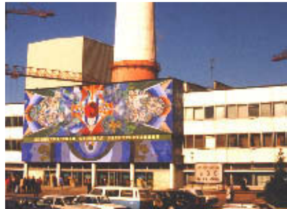
Figure 2-6: Entrance of Leningrad NPP (Photo: NRPA)
