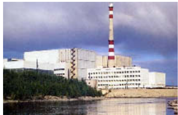
Figure 2-2: A view of Kola NPP (Photo NRPA)
